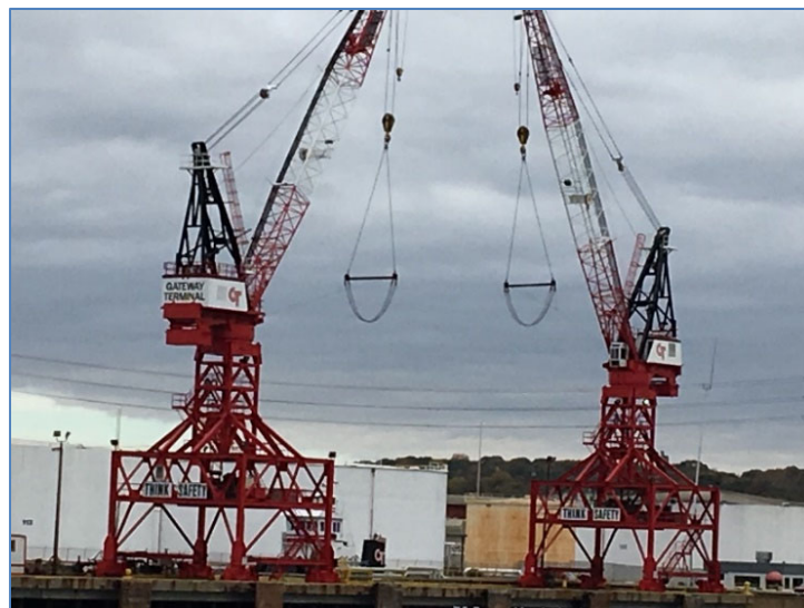
Figure 2-3c: Gateway Terminal Cranes
